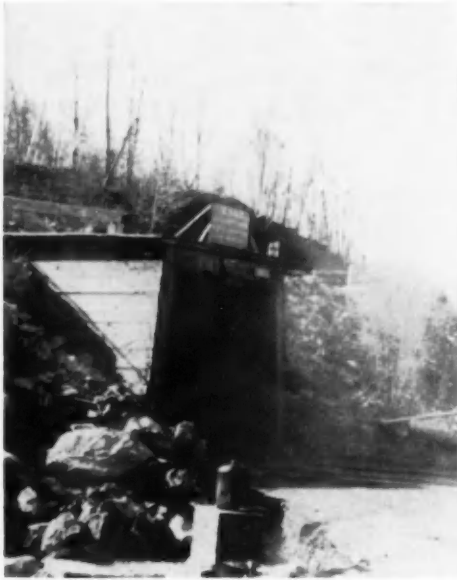
NEWEST TUNNEL ENTRANCE
